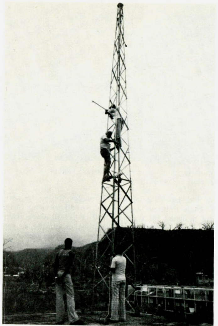
Photo U. J7DAY and KP2A, both up in the tower, erect home-brew antennas for use with the VHF gear sent by the IARU. They are assisted by VP2ABC, to the right, from a safer location. The tower was located on top of the police HQ building. In the background may be seen the devastated botanical gardens and a damaged school.
