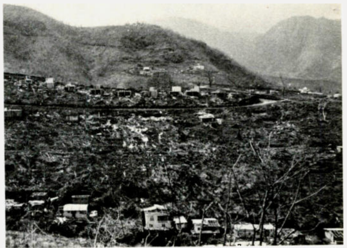
Photo G. View overlooking the Kingshill area, in the vicinity of J7DAY's QTH. There was nearly complete and total destruction of the houses in this area and to the south of Roseau.
