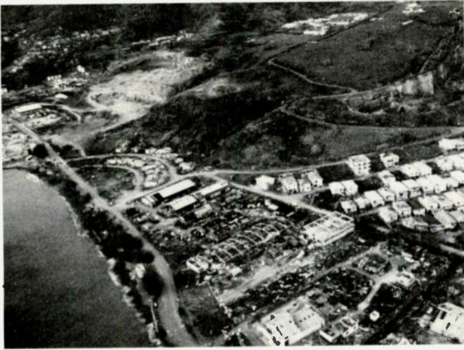
Photo F. Aerial photograph taken on Friday, August 31st, showing severely damaged warehouses on the outskirts of Roseau.
