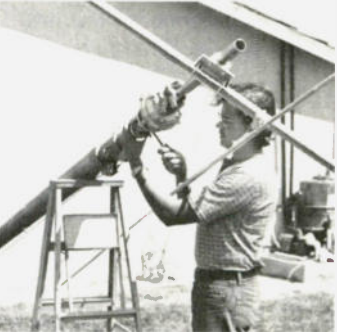
The Hinged Base Plate allows tower to be tilted over for access to antenna and rotor from the ground.
