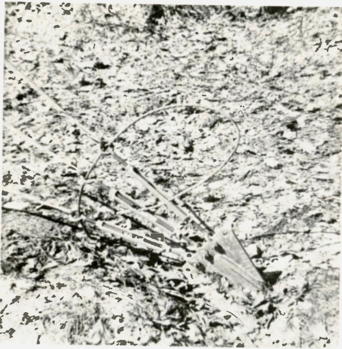
Here is a commercial tower anchor and "eyeplate." Note the length of guy wire laced through the turnbuckles to prevent loosening.
