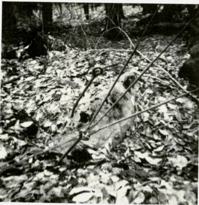
The anchor rod holds three guys using preformed grips. The rod is six feet long and is buried nearly five feet down.
