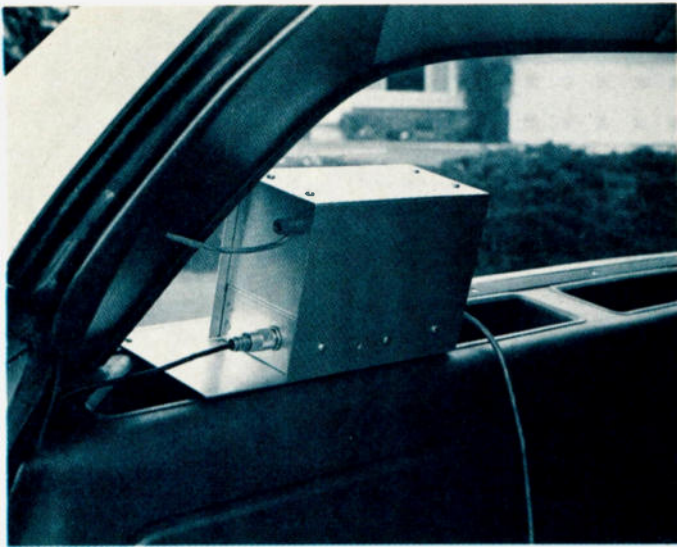
This neat installation of the tuning unit in the left rear window of my station wagon permits a short lead-in from the ball mount outside.
