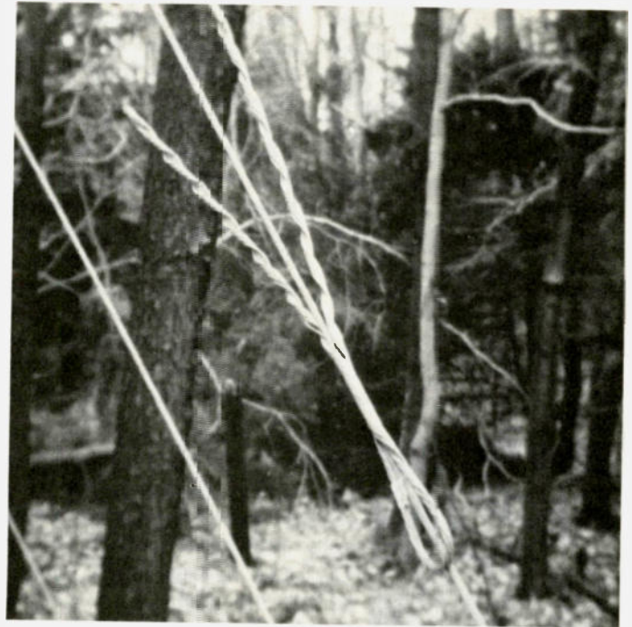
This is a partly installed preformed grip. No tools are needed, and it may be removed for re-tensioning of the guys and easily reapplied.
