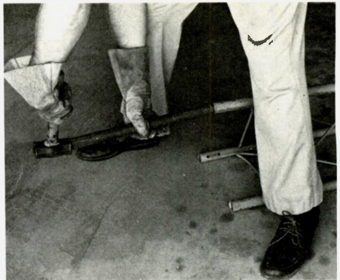
Photo F. Clearing excess galvanizing from the tower legs will make joining easier.
