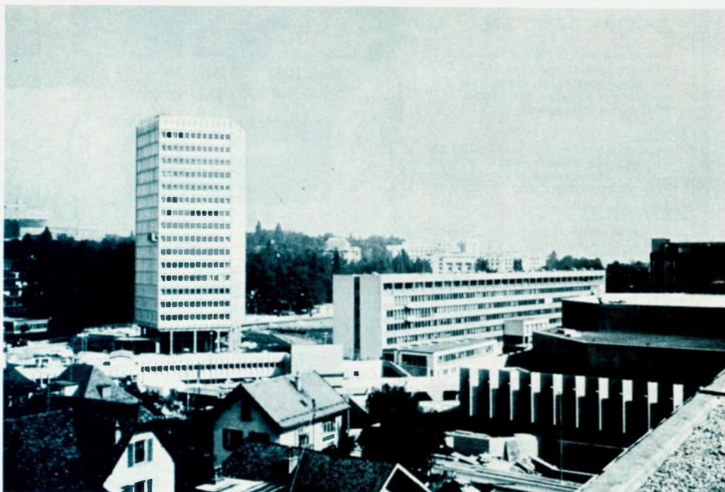
Headquarters of the International Telecommunication Union in Geneva, Switzerland.
