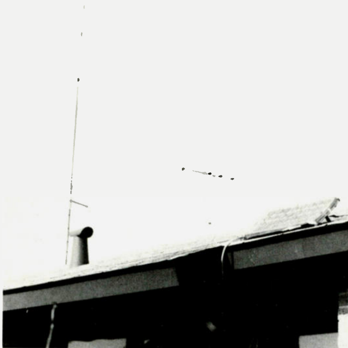
The multiconductor cable hanging from the left of the solar cell array is used to measure individual cell output, if desired.
