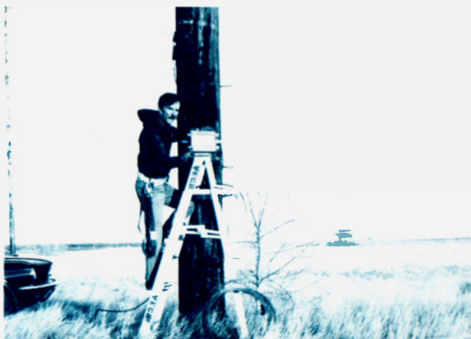
Installing the 1 kW broadband balun on the feed pole. The first two poles of my rhombic are used to support the beverage. The remaining poles are 20' long.
