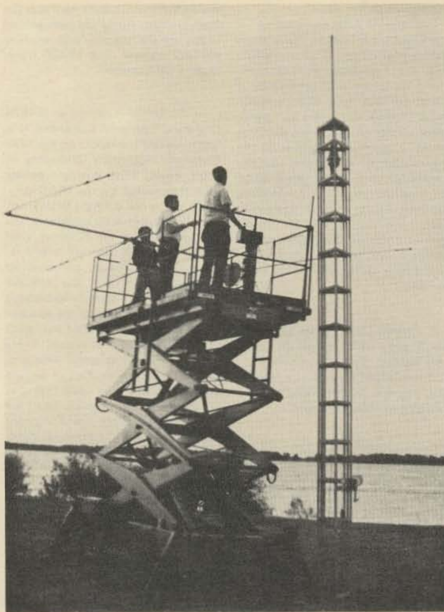
The extra effort separates the "serious" from the "enthusiastic." Here, the Dallas Amateur Radio Club effort illustrates the easy way to clamp a tribander onto a crankup tower. Thanks to the DARC.
