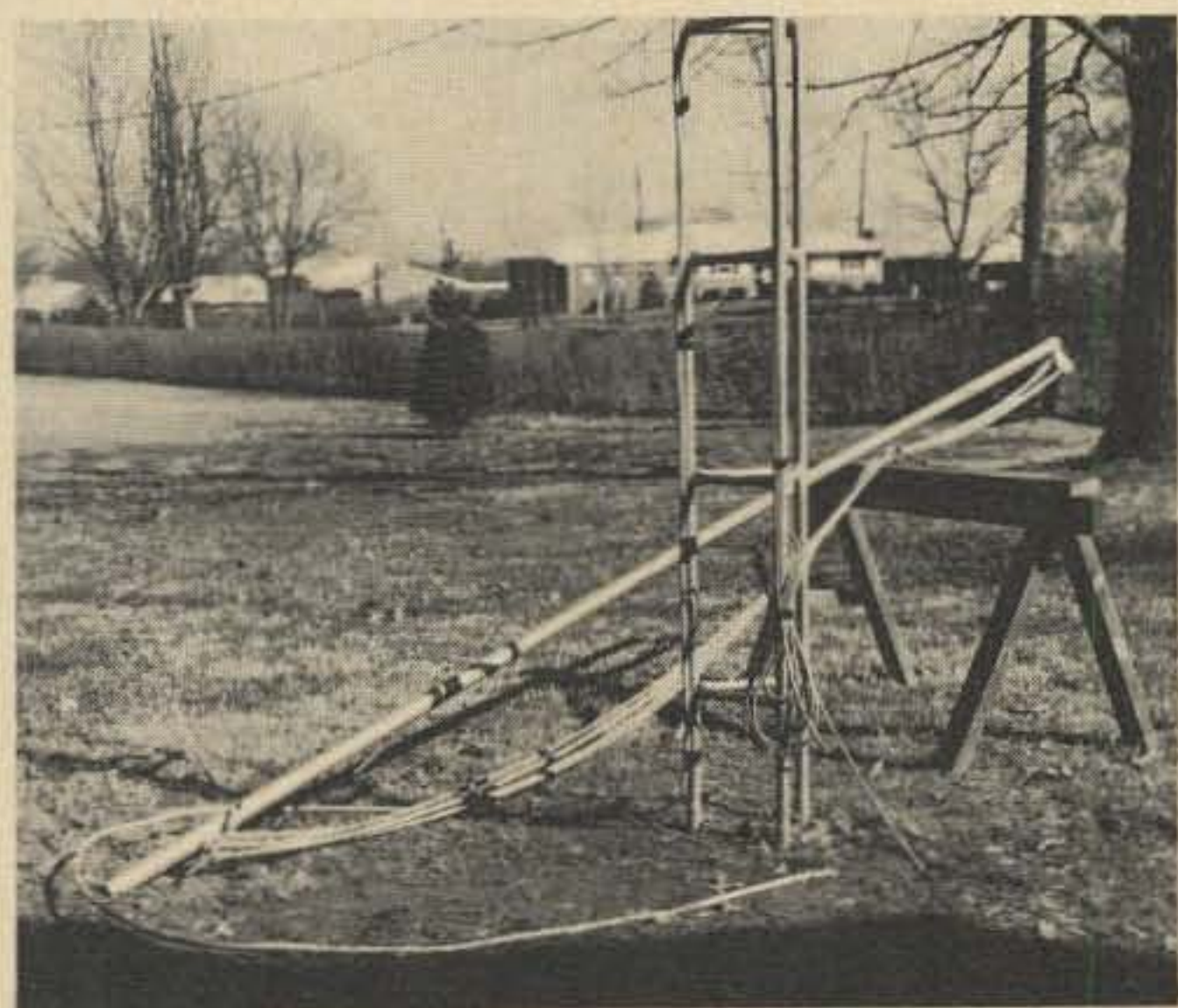
Fig. 7. The aluminum Foamflex transmission line (shown here above-ground) has been buried in a shallow trough; now I have a good crop of Kentucky bluegrass over it.
