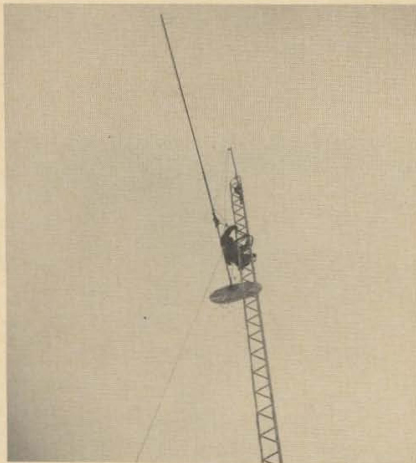
Fig. 3. Seen here is one of those crucial moments when "you don't know if he can make it but you don't dare ask!" Since this was a success with a 4 ft screen, a later modification to include a driven, reverse-phased aluminum element certainly made the job easier.
