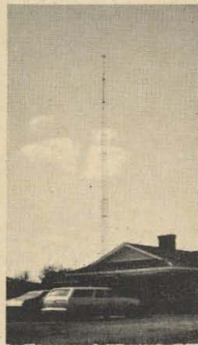
Fully extended Total tower height 69 ft.
