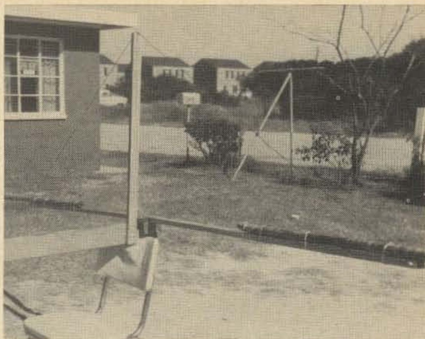
Detail of the element guy mast construction and use. Another set of guys is installed to a point about halfway down the length of each bamboo pole. See text for details.
