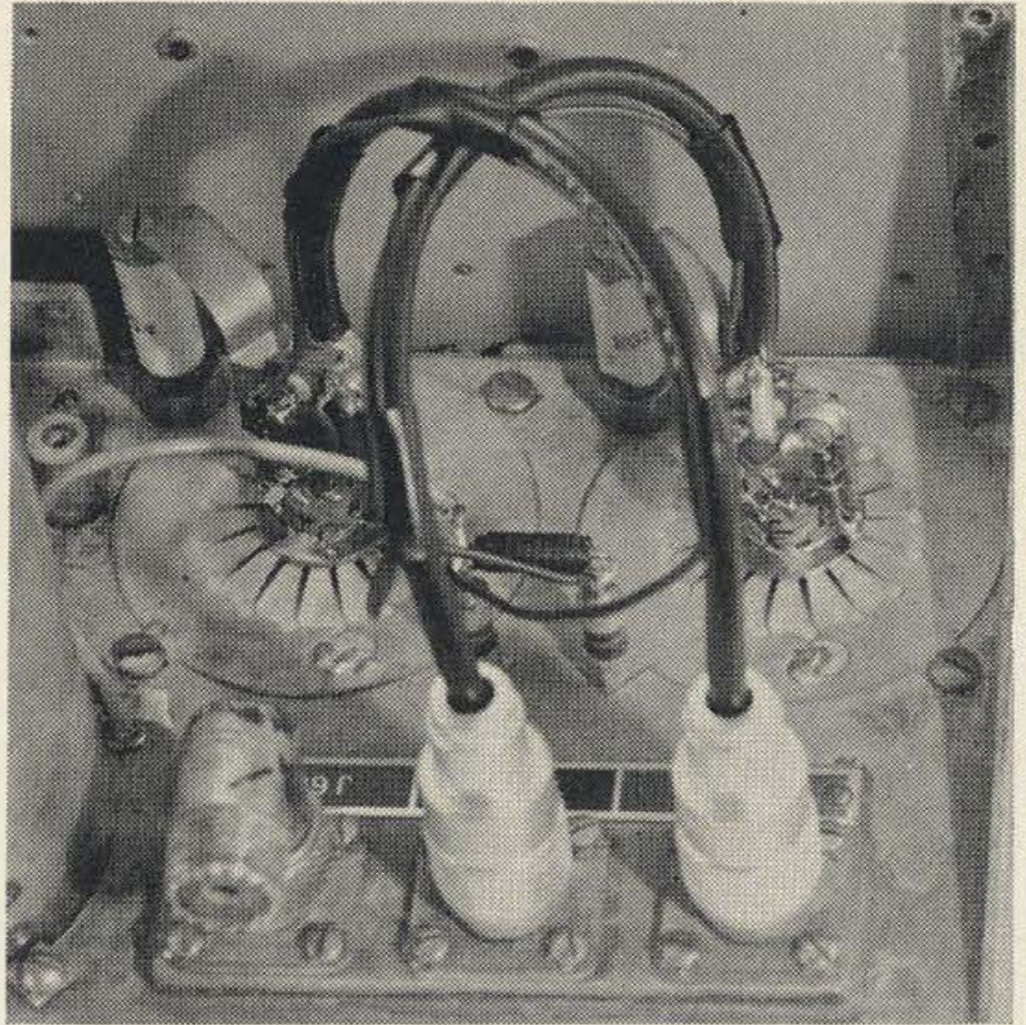
This photo shows the 8058 adapters plugged into the 46ADT chassis.
