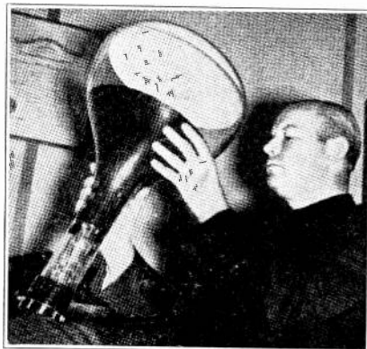
Fig. 262. Photograph of a large cathode ray tube such as used in some of the later type television receivers. This tube has a 12" diameter screen and is capable of producing television images similar to the one shown in Fig. 257. Courtesy DuMont Laboratories.
