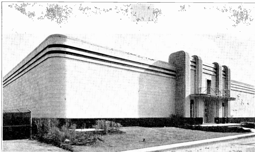
Fig. 158. This photo shows a modern air-conditioned building. Modern electric air-conditioning and electric lighting permit such buildings to be constructed without windows, thus shutting out noise, dirt, heat and cold very effectively. Courtesy National Aluminate Corp.
