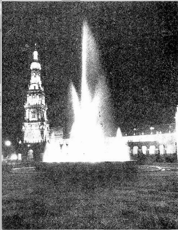
Fig. 216. The fountain in the foreground is illuminated by flood lights placed within its bowl, and in weather-proof projectors. In the background is shown a well flood-lighted tower.
