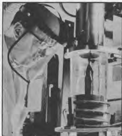
A physicist in the laboratories of Delco Radio inspects the growth of a large crystal of germanium which will be used to make many thousands of transistors. Germanium and silicon are the heart of most transistors and semiconductor diodes.
