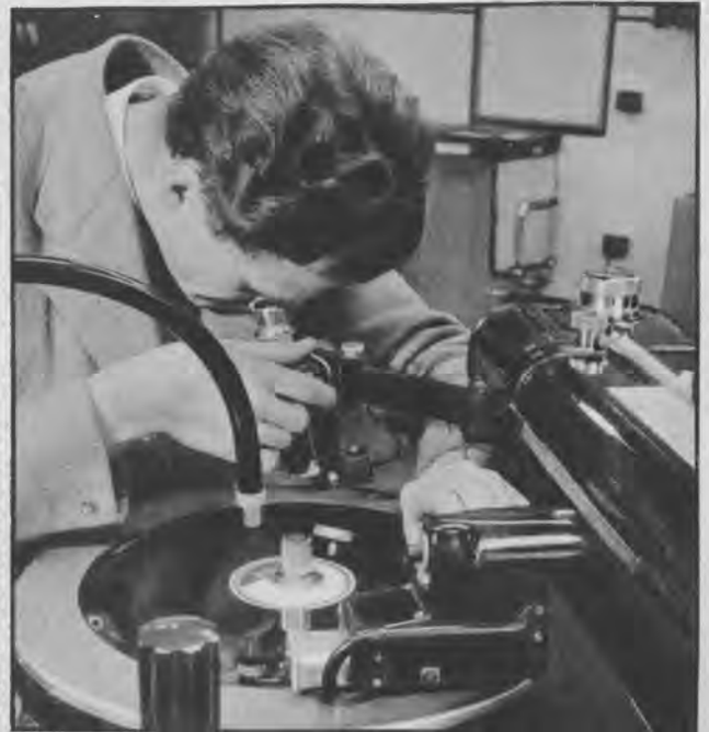
Figure 6: Taken from our files and somewhat dated, this picture nevertheless epitomises the care which goes into the preparation of a master recording. Here a B.B.C. engineer examines a test track with the aid of a permanent microscope and inspection light.
