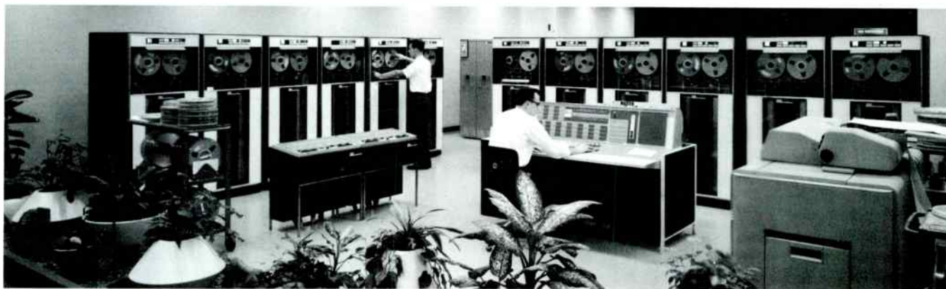
Photo Westinghouse computer center at East Pittsburgh.
