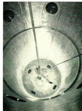
An inspector views the interior of the pressure vessel. Holes at bottom are inlets for primary water, those at top are outlets.
