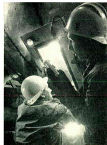
Workmen vacuum test welds on the reactor vessel thermal insulation.
