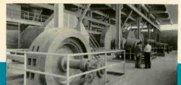
Huge ball mills are used for both raw and finish grinding.
