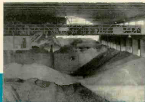
Ingredients for portland cement—both before and during processing—are stored in these huge bins.
