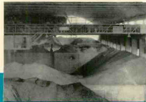
Ingredients for portland cement—both before and during processing—are stored in these huge bins.
