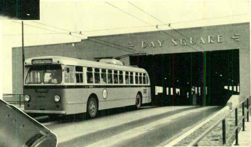
Fig. 1—Fifty-three new trolley coaches like the one shown above were placed in service in Boston recently. The electrical equipment in these coaches includes Super-Series d-c traction motors (inset) and Electrocams controllers.
