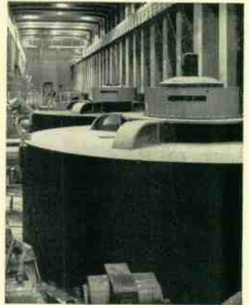
The Pump Motors , one of which is shown in the photo above, are 65 000-hp, 200-rpm synchronous motors rated at 13 600 volts, 3 phase, 60 cycles. They are direct-connected to single-stage, vertical-shaft, centrifugal pumps capable of lifting 700 000 gallons of water per minute.
