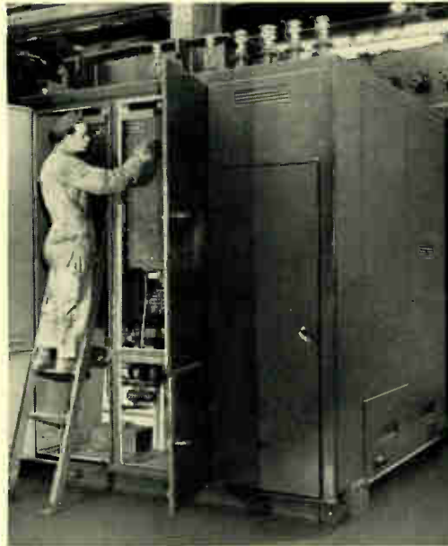
A CSP Power Transformer, rear and front views respectively, and the compartment at the rear of the circuit breaker.
