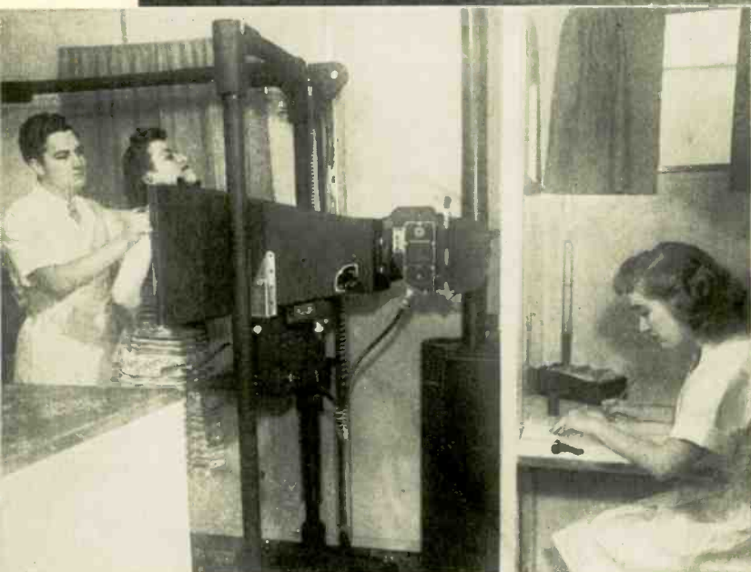
Truck trailers equipped with the photofluorographic x-rays are being used in a nationwide campaign to stamp out tuberculosis. The chest x-ray equipment uses small and inexpensive film, and is equipped for quick handling of large numbers of people. It also contains darkroom facilities.
