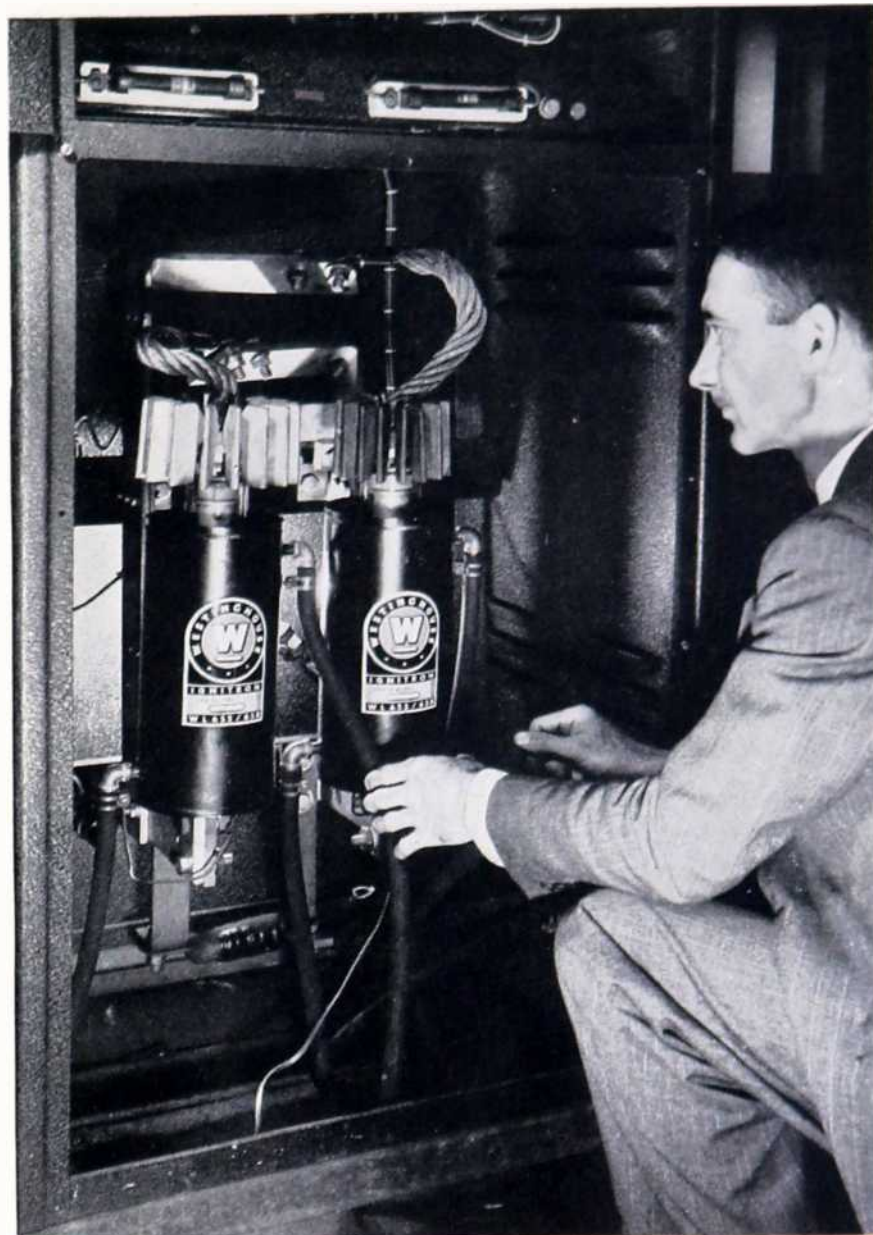
This pair of ignitrons is mounted in a cabinet for resistance-welding control. They each furnish 200 amperes at 440 volts for controlled periods of between two and thirty cycles.
