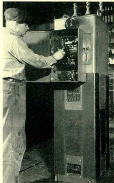
This air-cooled regulator is rated 48 kva at 2400 volts, four times the capacity and four times the voltage of the previous largest natural-draft air-cooled feeder regulator available (12 kva at 600 volts)
