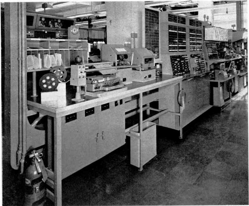
Figure 64. Central supervisory position
