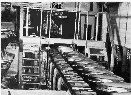
Photo 11—Color tubes' last mile of production is conveyed to exhaust machine.
