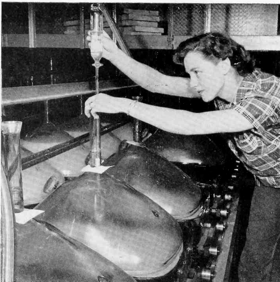
Figure 2. A controlled amount of lacquer is deposited upon the water cushion as the tube passes by on the belt.
