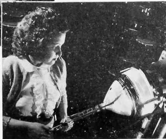
A Sylvania technician (above) is shown using one of the special glass lathes in one of the steps of the renecking process.
