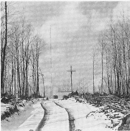
Figure 3. The KG2XDU tower and station building.
