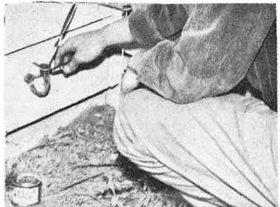
Fig. 67—Transmission Line Entrance
