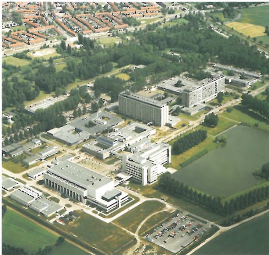
Fig. 14. An entirely new centre for studying and manufacturing ICs with details smaller than a thousandth of a millimetre — 'submicron details' — has appeared on the Philips Research Laboratories site in Eindhoven in recent years. The large building in the foreground is the pilot-production plant. The building behind it by the lake houses the research and design department.
