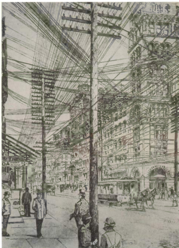
Fig. 1. At first, telephone connections were almost always made with overhead lines. Because there were so many wires, the result was not always particularly attractive. The picture shows a street scene in one of the larger cities in the United States in the early days of telephony (about 1880).
