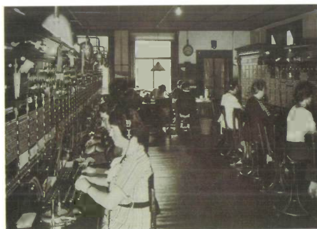
Fig. 9. An ordinary telephone exchange half a century ago (manual exchange, 1936).
