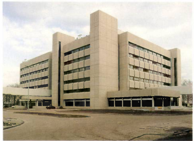
Fig. 2. The building where the circuits will be designed with the help of computers (CAD, Computer-Aided Design).
