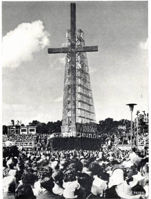
Fig. 13. Evangelical Church Congress, held on the Rebstock airfield near Frankfurt am Main (1956). In the vertical beam of the 40-metre high Cross, loudspeakers were mounted to form a sound column 30 metres long. The speaker on the platform could be clearly understood all over the ground, covering some 50 acres and on which a crowd of over 300 000 was assembled. At the end of the congress the installation was used for controlling the traffic.
