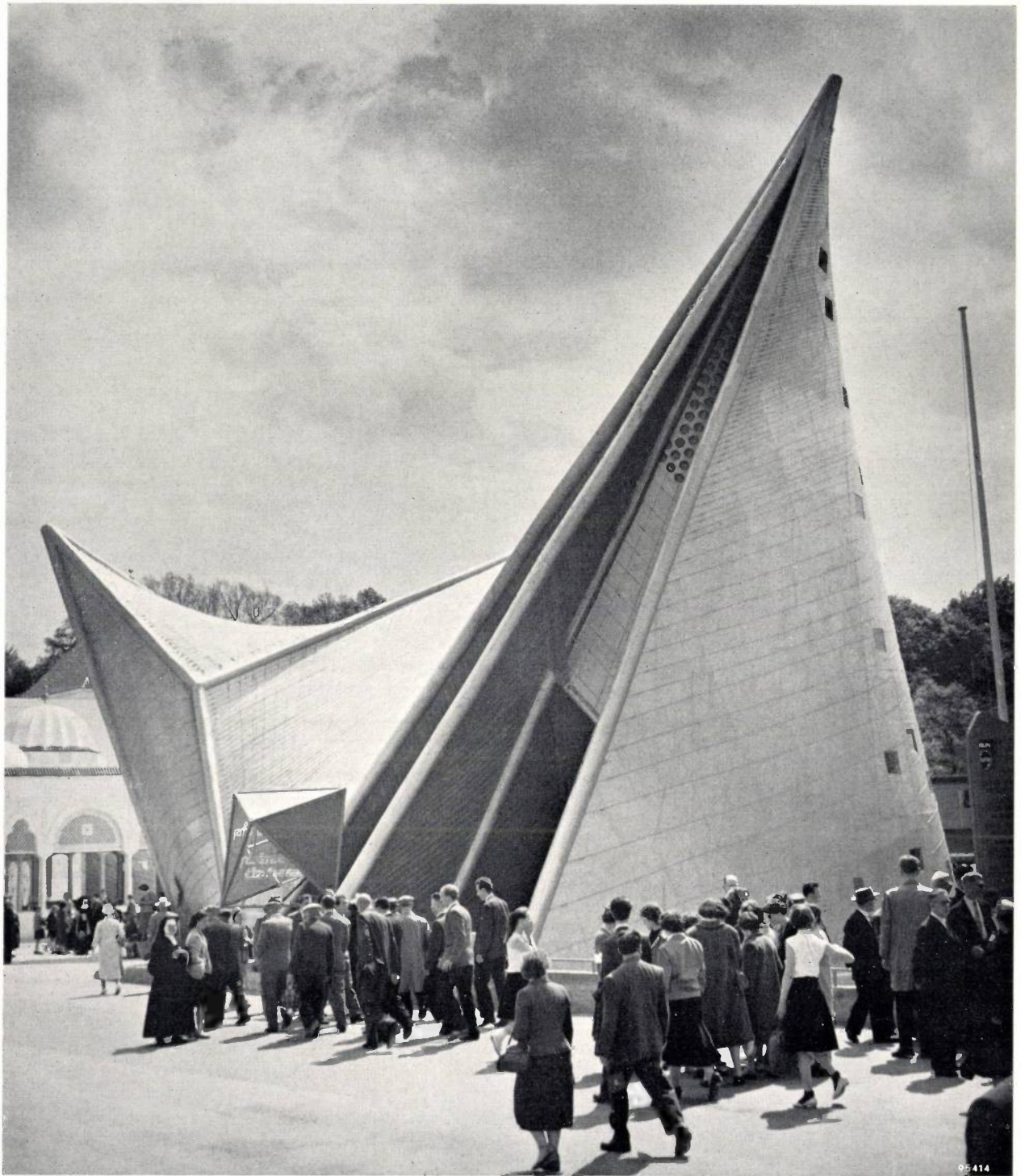
Fig. 12. The finished pavilion, seen from the entrance end.
