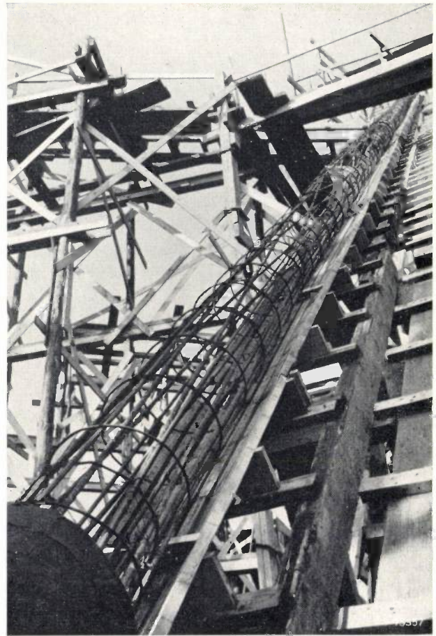
Fig. 9. Prestressing wires for a rib, mounted before making the shuttering and casting the concrete. This particular rib was fitted only with wires for producing torsional prestressing (eight wires running on the circumference of a cylinder, 35 cm in diameter, formed by a series of iron hoops). The 9 mm wires look thicker here since they have been coated with a preparation to prevent bonding with the concrete.
