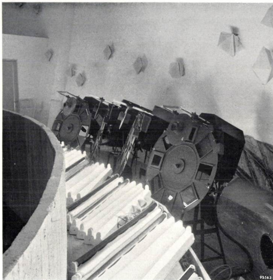
Fig. 5. Glimpse behind the balustrade. Some of the variously coloured fluorescent lamps can be seen and, behind them, an array of projection lanterns with filters for the "ambiances". Above, on the wall, a number of high-note loudspeakers. Bottom right a low-note loudspeaker.
