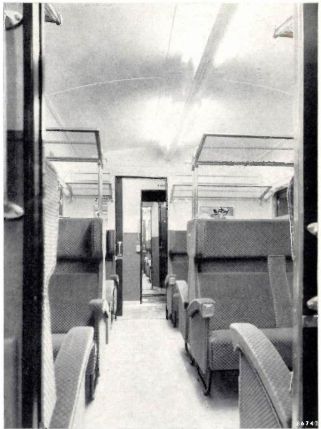
Fig. 13. Lighting in the carriage of an express train of the Netherlands Railways, using 40 W "TL" lamps, fed via a centrifugal converter.
