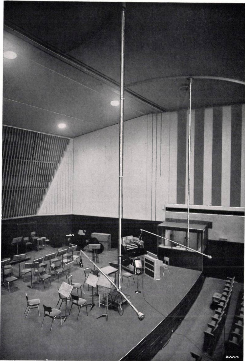
Fig. 2. Platform of the large concert hall in the A.V.R.O. building. Two suspended microphones hang from rails in the ceiling along which they can be moved in order to be able to place the microphones as nearly as possible at any desired spot. In the background may be seen the mixing cabin which is separated from the hall by triple glass windows.
