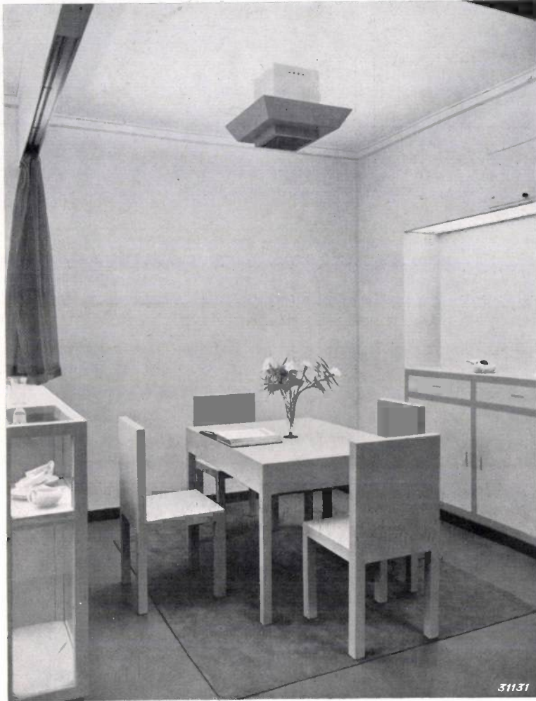
Fig. 8. Dining room. Indirect illumination with four "Cornalux" lamps of 60 W. Illumination above the sideboard by five lamps of 25 Dhm above a plate of frosted glass. Direct illumination, directed on to the table, from a mirror reflector "Philiray" SC 255 with an "Argenta" lamp of 200 W. The average intensity of illumination on the table is 250 lux. This light is not on in the photograph, but it may be seen in fig. 1.
