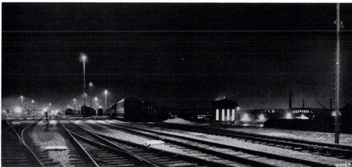
Fig. 7. Railway yard, Dijkgracht, Amsterdam, lighted with 39 "Philora" sodium lamps SO 85 W. The height of the light points is 10.5 m.
