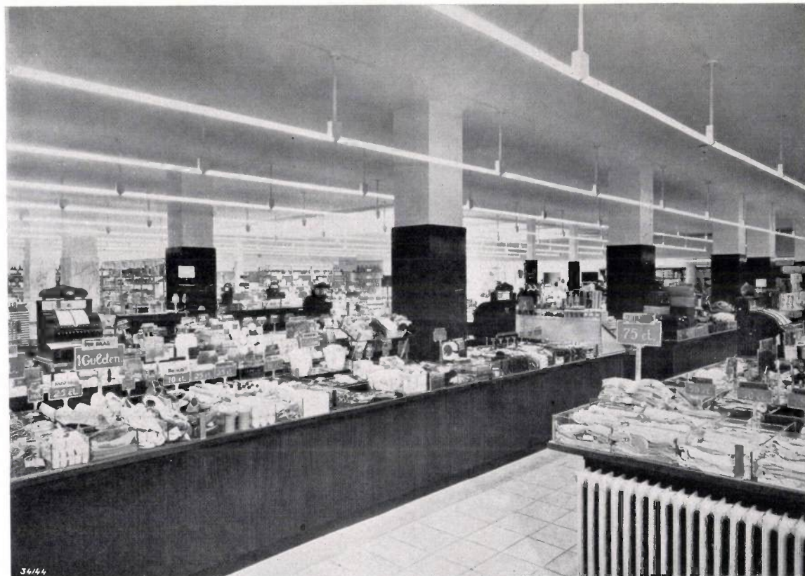
Fig. 3. Installation of a series of luminescence lamps in a shop.
