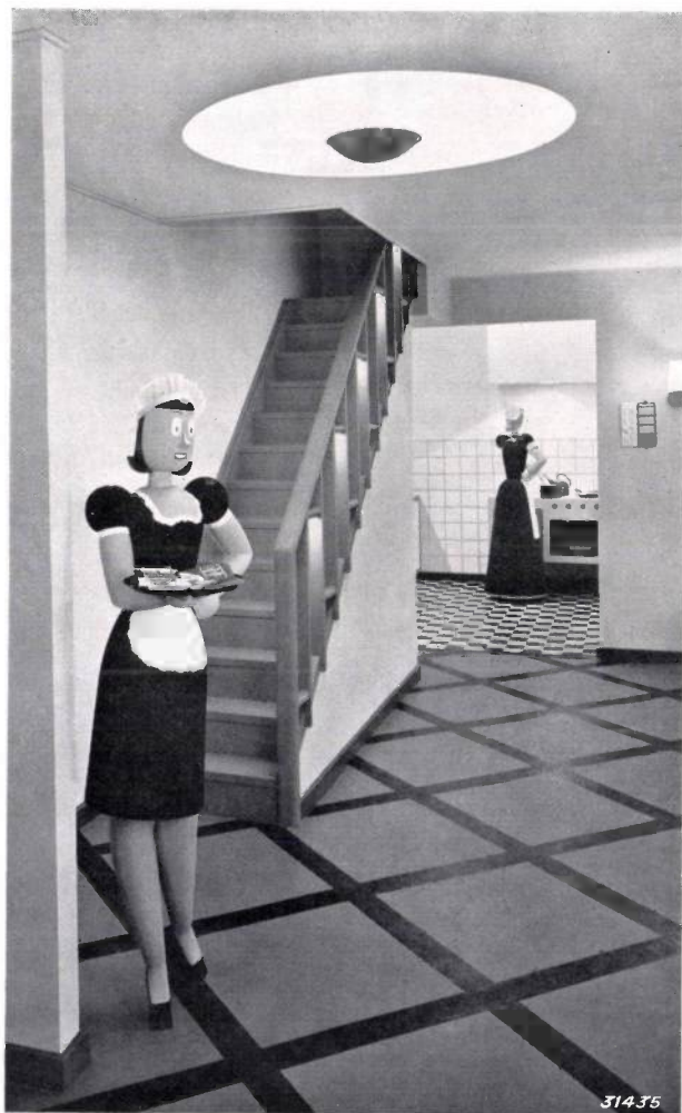
Fig. 3. Hall of the "well lighted house", seen from the bathroom. In the background the kitchen. The treads of the stairs are lighted by lamps built in at the base of the bannister. The dummy figures in this house were designed by George Pál.
