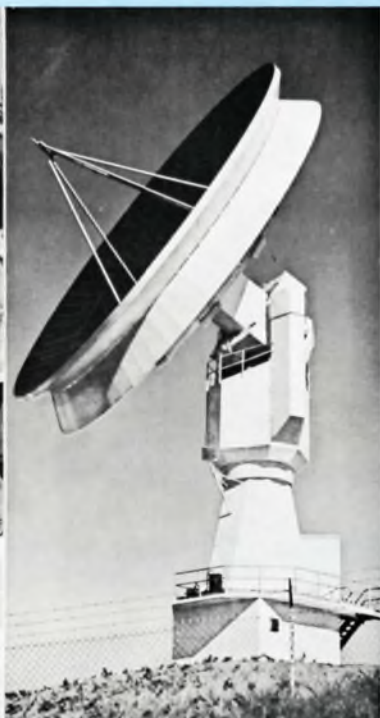
How do you get information from a satellite in space? In any phase of flight there's a big problem. How do you track a satellite or something like that? Philco-Bendix designed and built the Philco satellite tracking antenna. This satellite tracking antenna and complete equipment are complete facilities of command, control, communication, receiving. Standing 80 feet high, with a 50-foot diameter antenna, it is the largest antenna of its kind in the world.
