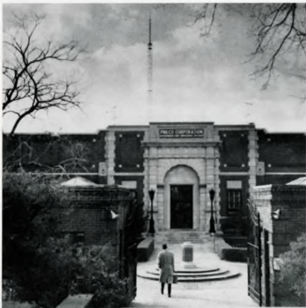
PHILADELPHIA'S LATEST TV BROADCASTING STATION—KG2XCV—is using this 150-foot antenna atop Philco's Government and Industrial Division Plant at 4700 Wissahickon Avenue. The Division is operating the experimental UHF station on Channel 23 for development of equipment.
