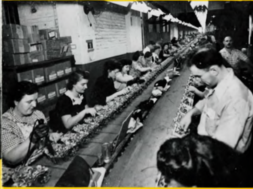
3 TEST MOUNTING —Full electrical tests are given the automobile radio sets to insure Philco quality. James Prendegrast has supervision of this operation and that of packing. ▼
