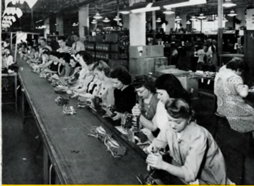
1 HEAD ASSEMBLY —Push-button and tuning controls are mounted to ▲ the wiring chassis on this belt in Dept. 86. Clayton Ziegler supervises the work on this line.
