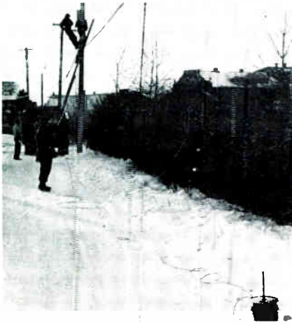
Line crew mounting ADO-10 box on pole, distance from the nearest television station.
