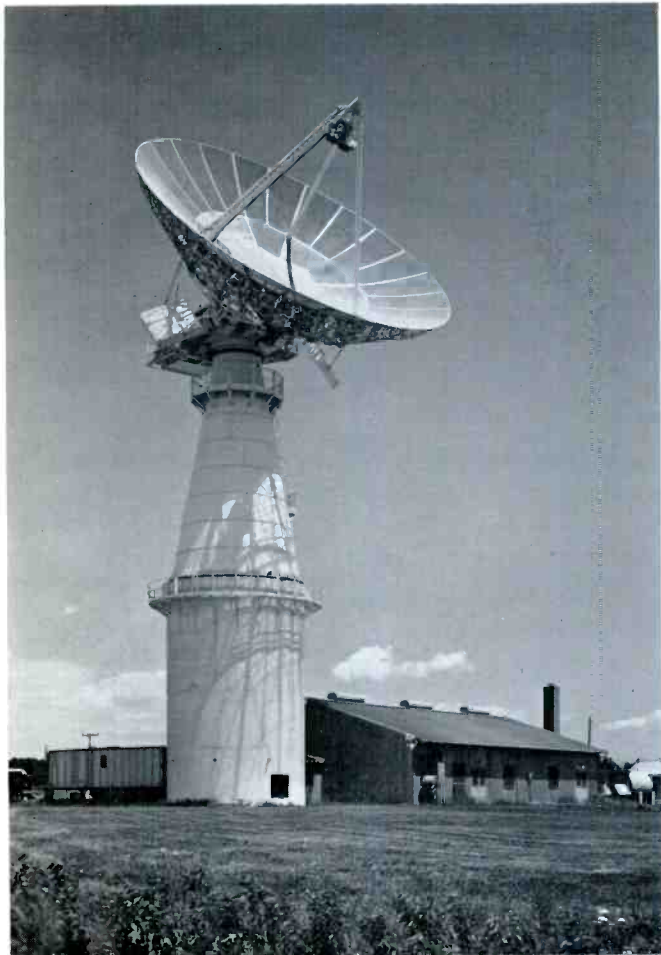
Figure 1 — NASA's SPANDAR, long range tracking radar, at Wallops Island, Virginia, employs a Raytheon designed, constructed and installed radar transmitter using the ML-7560 as a modulator switch tube. Shown here are the 60-foot parabolic antenna and 90-foot tower of the installation.
