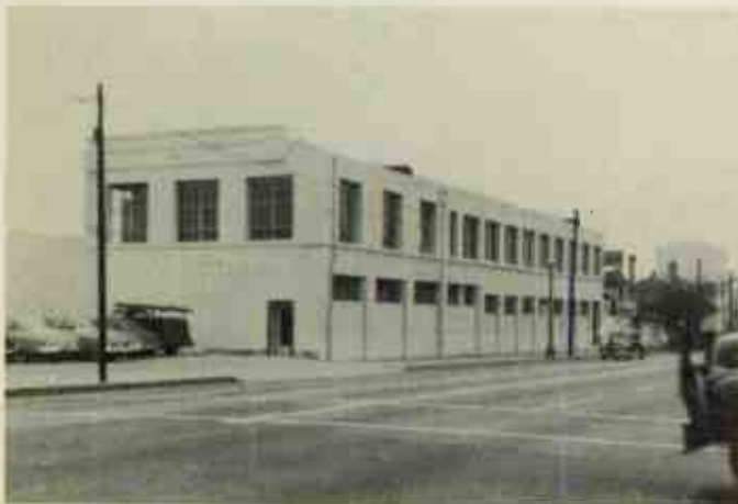
View of the new building looking south from College and Castelar.
