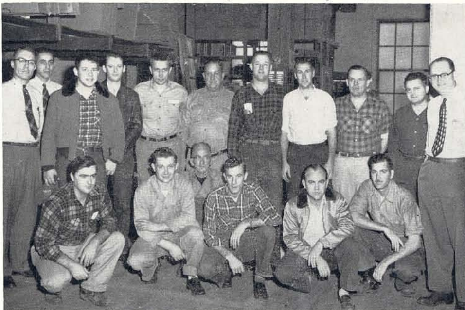
Members of Fire Committee and the areas they represent are pictured above. Kneeling from left to right are: Don Hubbard, Test Laboratory; Gib Allen, Shipping; Turk Hill, Stock Warehouse; John Harrison, Cable Department; Charles Bridgman and Art Miller, Sheet Metal. Standing from left to right are: Personnel Director, Rog Veach; Industrial Engineer, Jack Eliason; John Maxwell and Jim Gibson, Rhodes' Assembly Department; Mel Arns, Stock; Tony Lohman, Foster's Assembly Department; Kyle Snowhill and Gene Crossan, Bonness' Assembly Department; Harold Laws, Engineering Development; Weldon Steinbach, Engineering; and Plant Manager, Howard Young.
