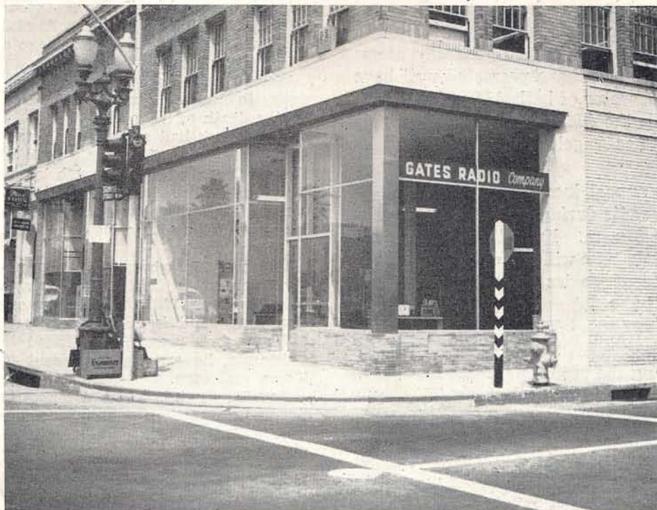
Front view of the new Gates Factory Branch located on Sunset Blvd. in Los Angeles, Calif.
