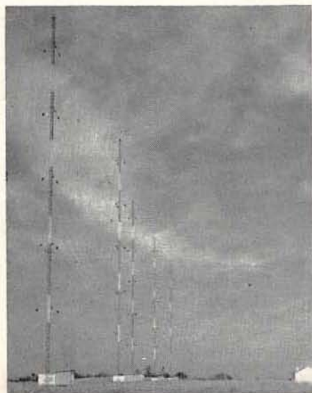
The associated five-tower phasor gives a real wallop to spread the signal over the southern tier section of New York State.
