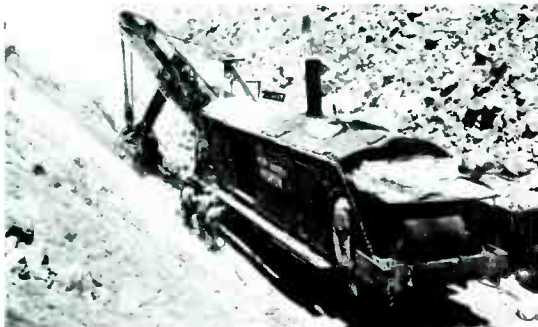
Steam-powered shovels, mechanical marvels of the early 1900s, replaced the pickaxe and hand shovel.
