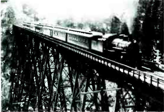
Utah's railroad construction included trestles, tunnels, bridges, grading, ballasting and track-laying.
