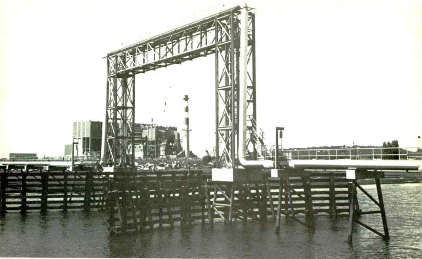
Steam pipe over the Saugus River links GE plant with RESCO facility visible in background.
