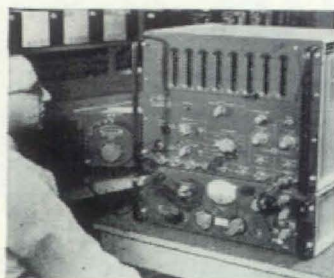
Development Engineer H. T. McAleer measures the frequency stability of a Type 1215-B Unit Oscillator at 250 Mc with the Type 1130-A Digital Time and Frequency Meter and the Type 1133-A Frequency Converter.
