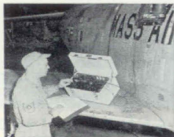
The Type 1429-A Fuel-Gage Tester (TTU-68/E) in operation at an Air National Guard Base.
