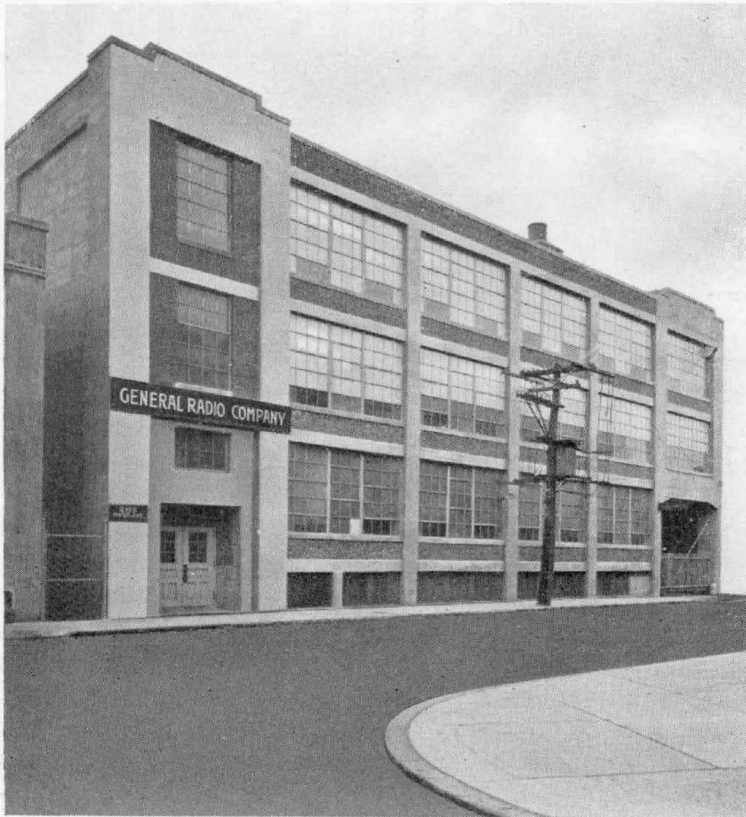
Building No. 1, erected 1924. Building No. 2 which was erected in 1925 is similar to No. 1 but is one story taller. Building No. 3 now under construction is similar to Building No. 2
