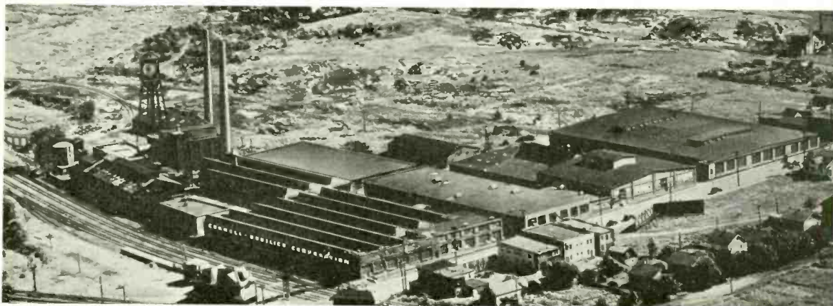
THE NEW PLANT OF THE CORNELL-DUBILIER CORPORATION AT SOUTH PLAINFIELD, NEW JERSEY.
