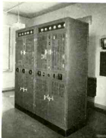
THE 1-KW TRANSMITTER.
