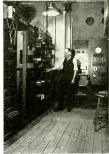
THE TELEVISION CONTROL ROOM.
