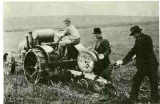
THE SPECIAL PLOW USED FOR LAYING THE GROUND WIRES.
