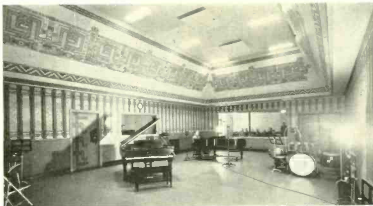
STUDIO "A"—ONE OF THE NEW SOUNDPROOFED STUDIOS OF KDKA WITH FLOATING WALL CONSTRUCTION. NOTE FRESH AIR SPLAYS ON CEILING, ALSO FLUSH LIGHTING FIXTURES.
