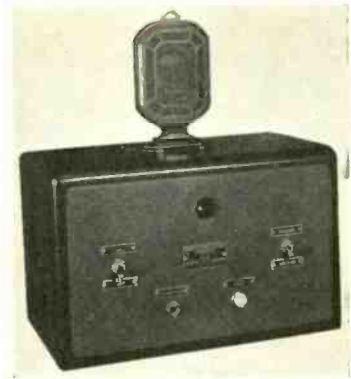
FIG. 4. CONTROL BOX FOR ET-5017 TRANSMITTER.
