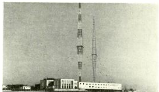
Fig. 1. A view of “Radio Vienna.” The transmitter is housed in the central building. The building on the right is the home of the technical staff.
